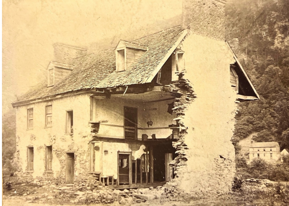
A recently-discovered cabinet card photo shows what is believed to be Phillip Coons' Butcher Shop and Boarding House on Virginius Island following the 1889 flood.
